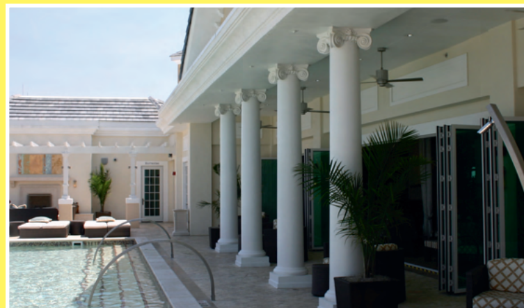
Photo right shows the use of Spectis columns with Scamozzi caps and Tuscan bases, custom moulding and custom trellis system
