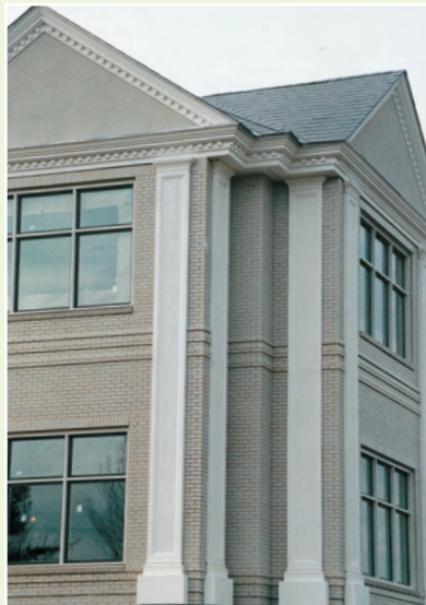
26' Tall Exterior Pilasters
