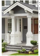
Spectis Moulders offers four different styles of PVC Box Column Wraps to beautify an existing structural post.
